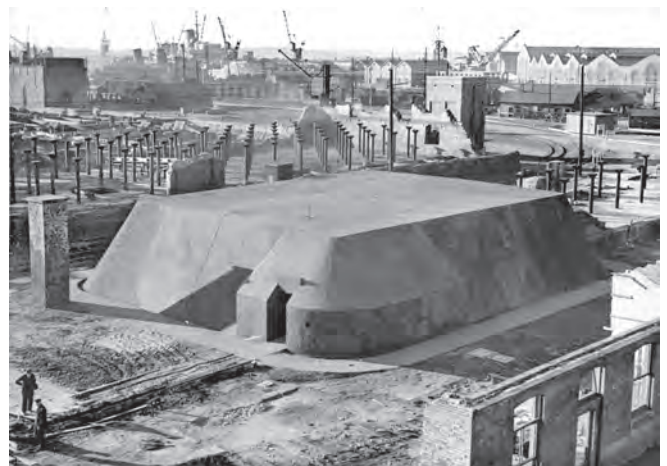
The completed bunker seen from the northeast. The entrance to the Southampton Docks control room is seen on the corner. The remains of the M warehouse are seen behind the bunker
